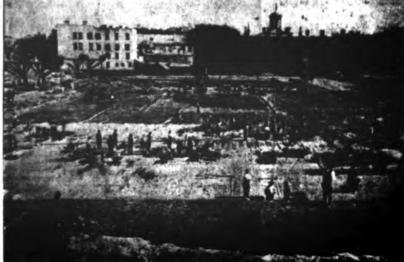
Covering approximately two acres with a foundation capable of supporting the weight of one of the world's most pretentious capitol was an arduous task...
