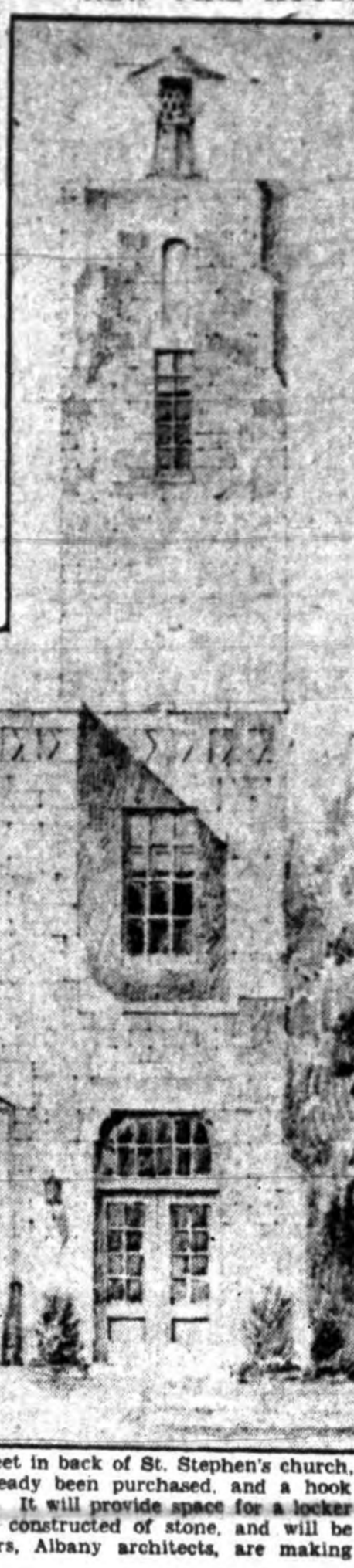
The new Elsmere firehouse which is to be erected on Herber street in back of St. Stephen's church. The building will house a pumper, which has already been purchased and a hook and ladder, if such apparatus is found to be necessary for the town. It will provide space for a locker room, showers, dressing rooms, meeting rooms and office. It is to be constructed of stone, and will be fifty feet in length, and thirty-six feet in width. Pember and Demers, Albany architects, are making the plans.
