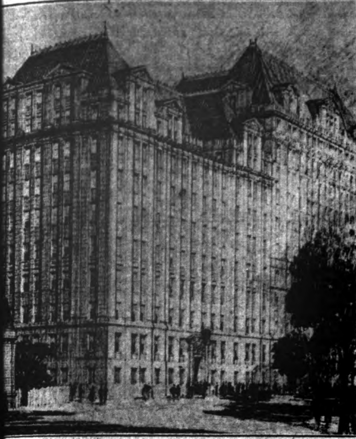
Architect's conception of the way the new addition to the New York Telephone company's building when completed. The addition is directly behind the main structure at 158 State street and 170 feet from the rear line of the present building along Park street and will have a front facade of brick and stone, conforming with the present building. The building is to be nine stories above ground level. The foundation work is practically completed and the erection of steel has started. The outside of the building will be of brick and stone, conforming with the present building. It is to house additional equipment and provide more office space for the company.
