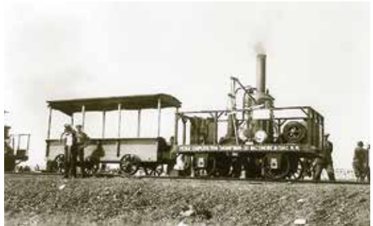
By 1830, Peter Cooper, an inventor from New York, completed work on his revolutionary invention for replacing horsepower with steam. The Tom Thumb, an experimental steam locomotive, never got beyond the test stage, but it paved the way for more advanced locomotives.
