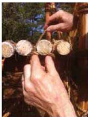
Looping bight over floor spar
