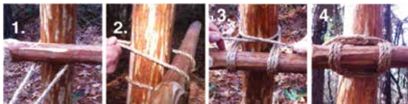
Straightforward approach for lashing two poles together
