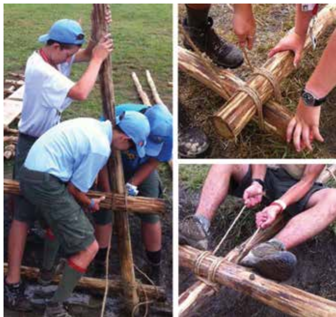
Straightforward approach for lashing two poles together
