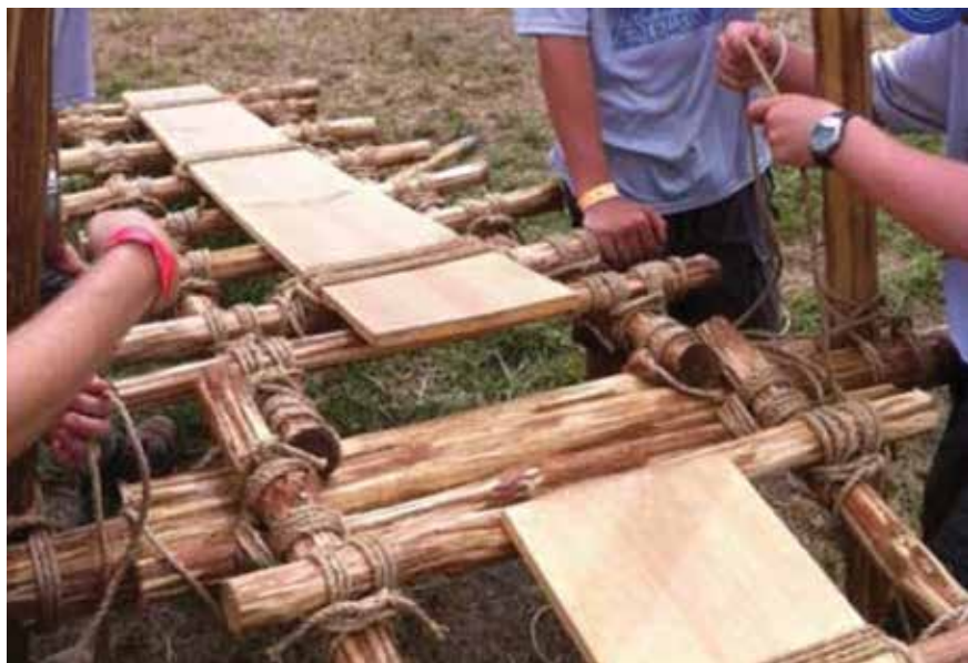
Joining the underspars of the walkways to the trestle's transom
