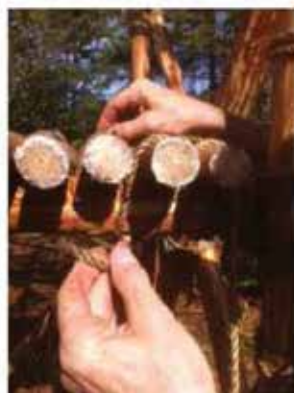
Passing it under platform support
